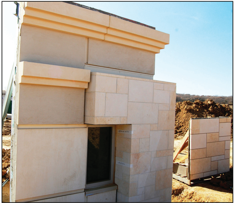
FIGURE 1.16 A typical mockup showing various finishes on the exterior facade of a building under construction. The workmanship in the finished building will be evaluated to match that of the approved mockup.
