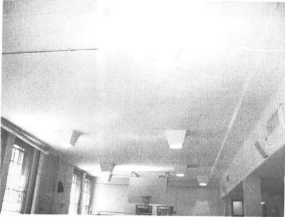
X046 Ceiling After 3
