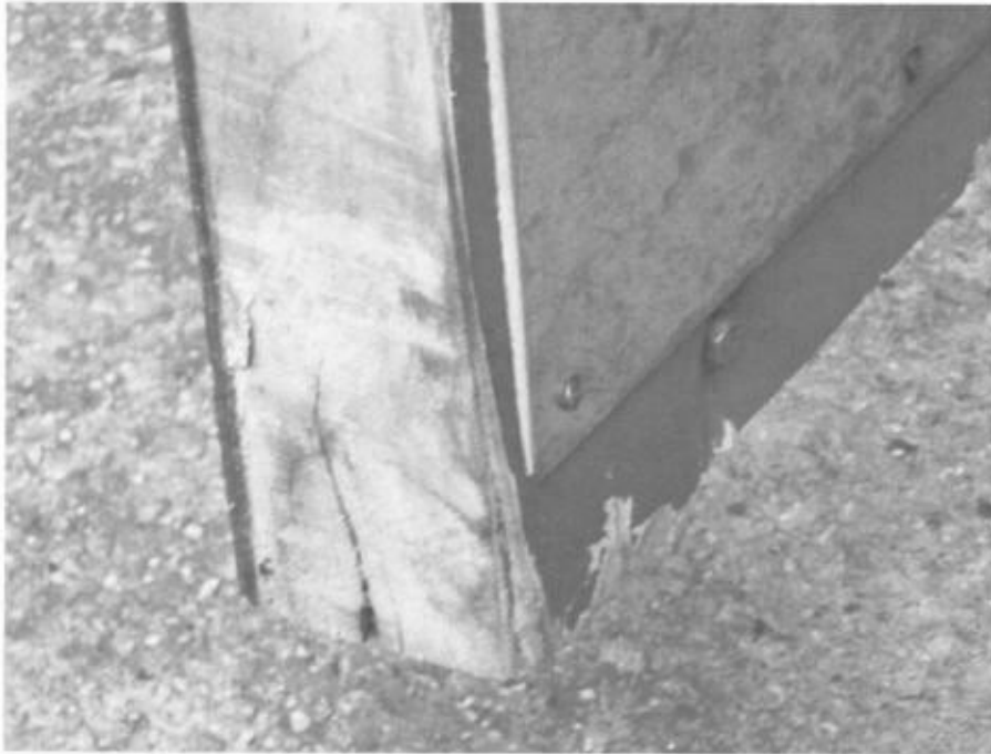
PS 70 Queens, Photograph #2, Exit Door Corrosion
