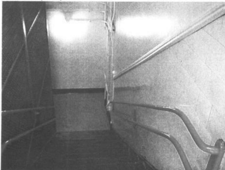
K138 Wall (After)
