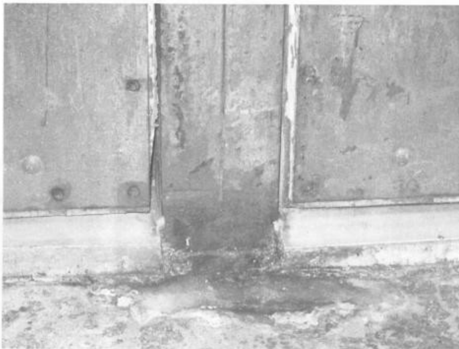
PS 70 Queens, Photograph #2, Exit Door Corrosion
