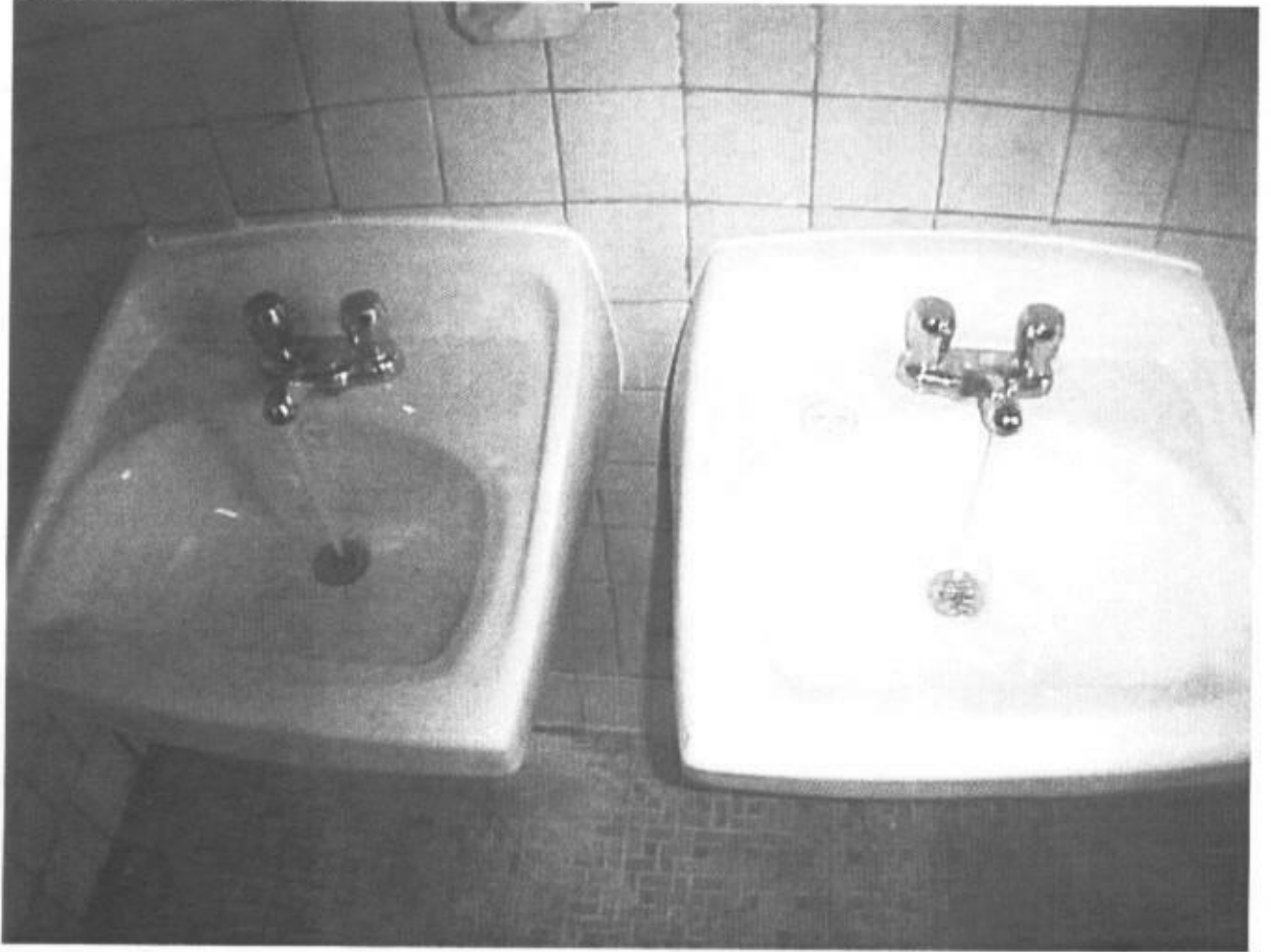
K028 Faucets Installed
